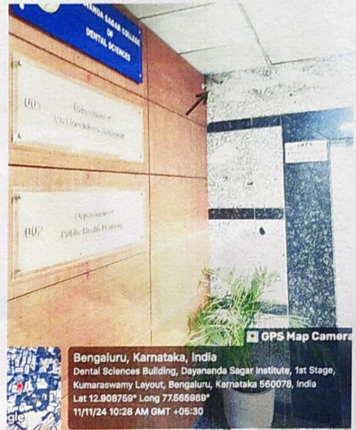
CCTV camera near the lift
